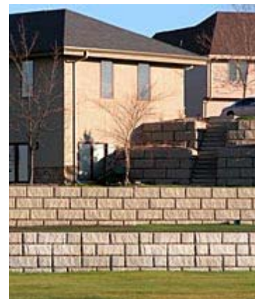
Commercial pavers hold back a lot of earth in residential landscapes.
